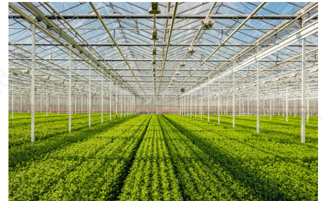
Agricultural Greenhouse Structures
