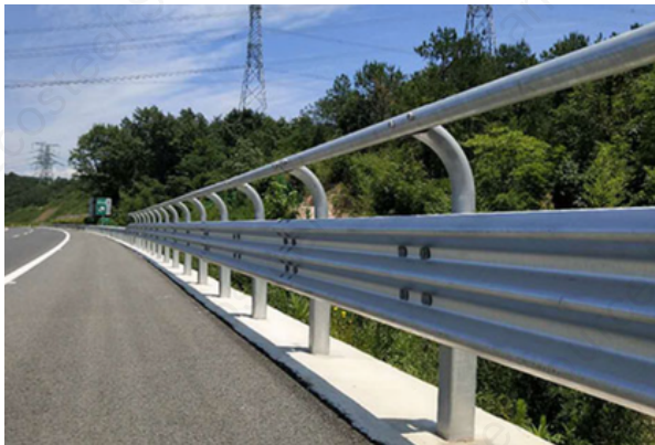
Guardrails and Highway Barriers
